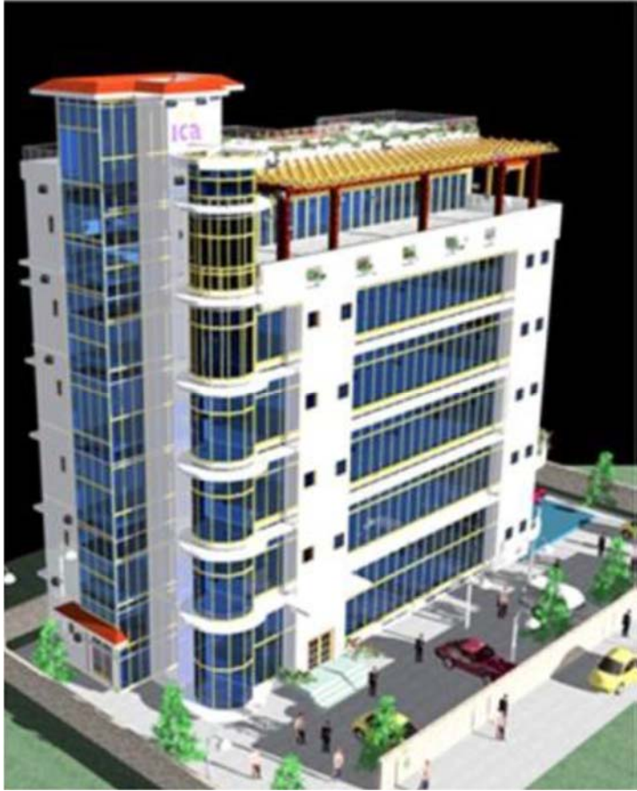
Office Building, I.C.A. Domus Trust Noida
